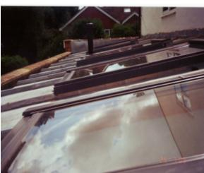
To the side: the kitchen joined up with the utility & additional living space. This required four veluxes seating within a zinc mono-pitch roof and two lead valleys to carry the rainwater behind a new tile mansard.
