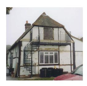
Roughcasting & sand/cement rendering were carried out in order to match the original external finishes. This photo was taken halfway through the project in 2004 that was completed on time, to budget with no recalls.
